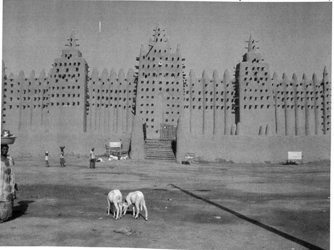
Great Mosque of Djenné, Mali. The first recorded mosque on this site was built in the thirteenth century CE. Made entirely of mud brick, it has been periodically repaired or rebuilt; the present structure was erected in 1907.
