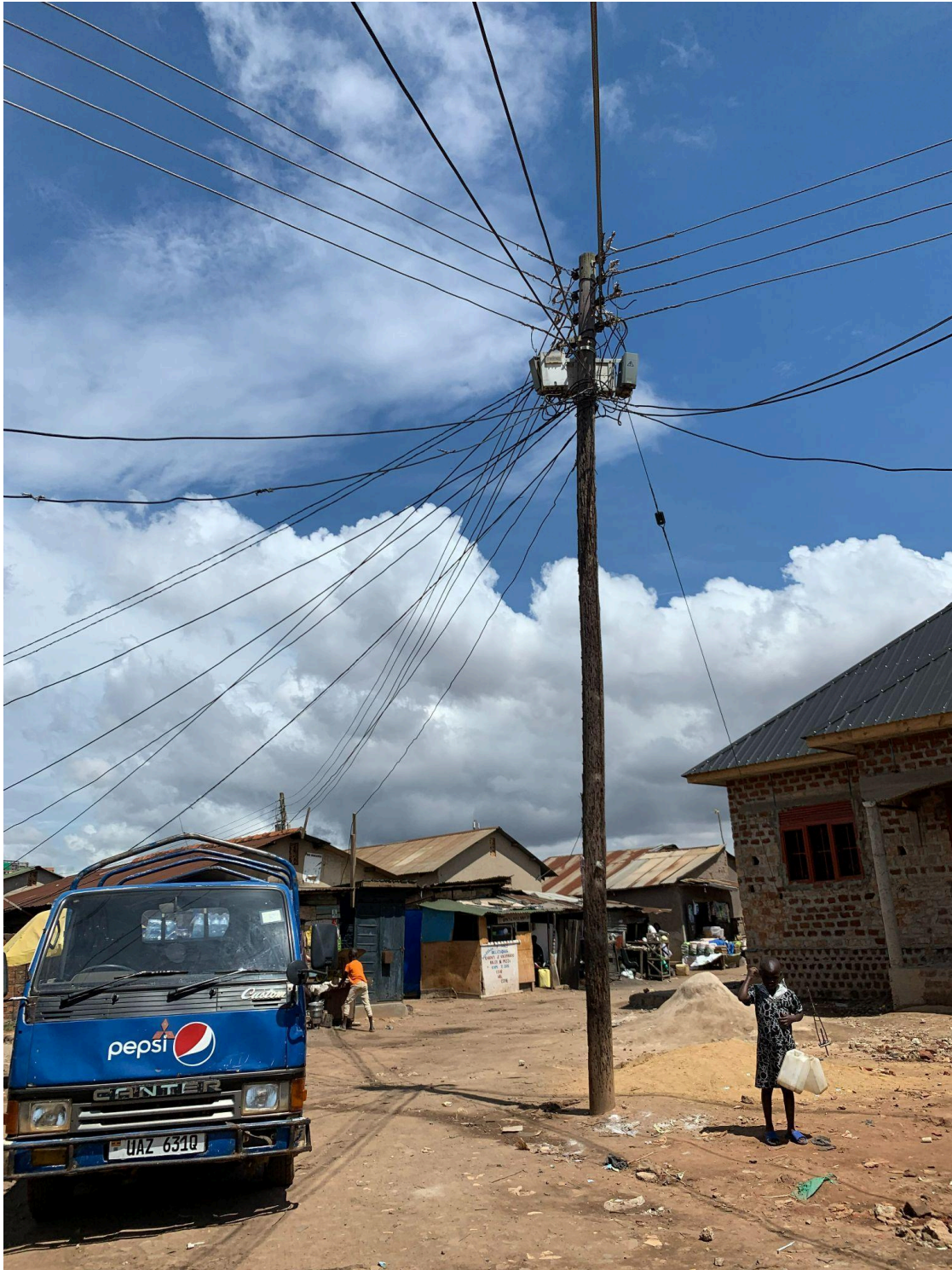
Photo 6. An LC leader pointed out this utility pole, commenting that “the tree [pole] is tired.” He is referring to the damage to the pole from kamyufus and utility workers, who use spiked metal boots to climb them and access the meter boxes at the top. On the pole, it is noticeable that the number of service lines is much greater than the number of meter boxes. These could be abandoned lines, but are more likely to be unmetered connections.
