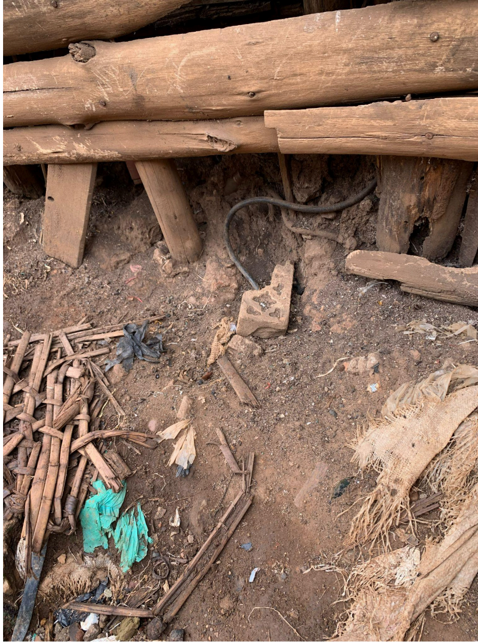
Photo 11. An electricity cable emerging from the ground and entering the wooden home above. This is also a footpath, and the concrete block was likely placed over it to protect it from bypassers, and vice versa. Undergrounding is the best way of disguising an illegal connection, but is dangerous. Several interviewees noted that underground cables like this used to cause several fatalities per year, but this practice is now less common. As one kamyufu explained, “If a wire gets damaged and is exposed especially in this place that floods when it rains, we have to be careful and advise [people] to switch off electricity when it rains, because this water can even kill people so we strive hard to switch it all off when it rains, and connect back when it stops.”
