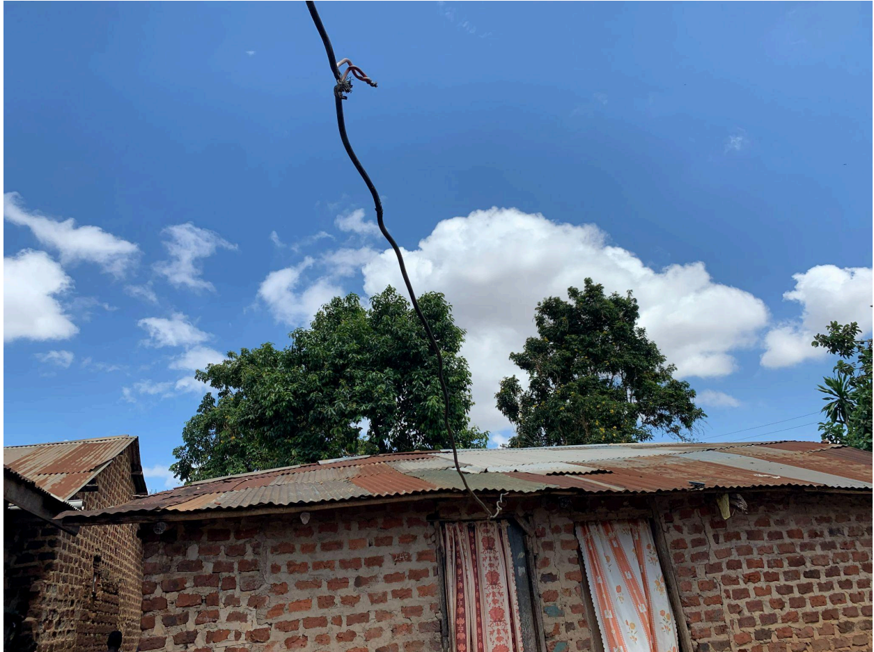
Photo 7. A household connection with a bare splice in the line. It is possible that this was done intentionally to make the line easy to disconnect. This might be done by a kamyufu , for example, so that the line can be concealed in the case of an enforcement raid by the utility and law enforcement. The ability to easily disconnect might also be desirable for landlords, who tend to use electricity as leverage and often cut the electricity supply if rent is not paid on time.
