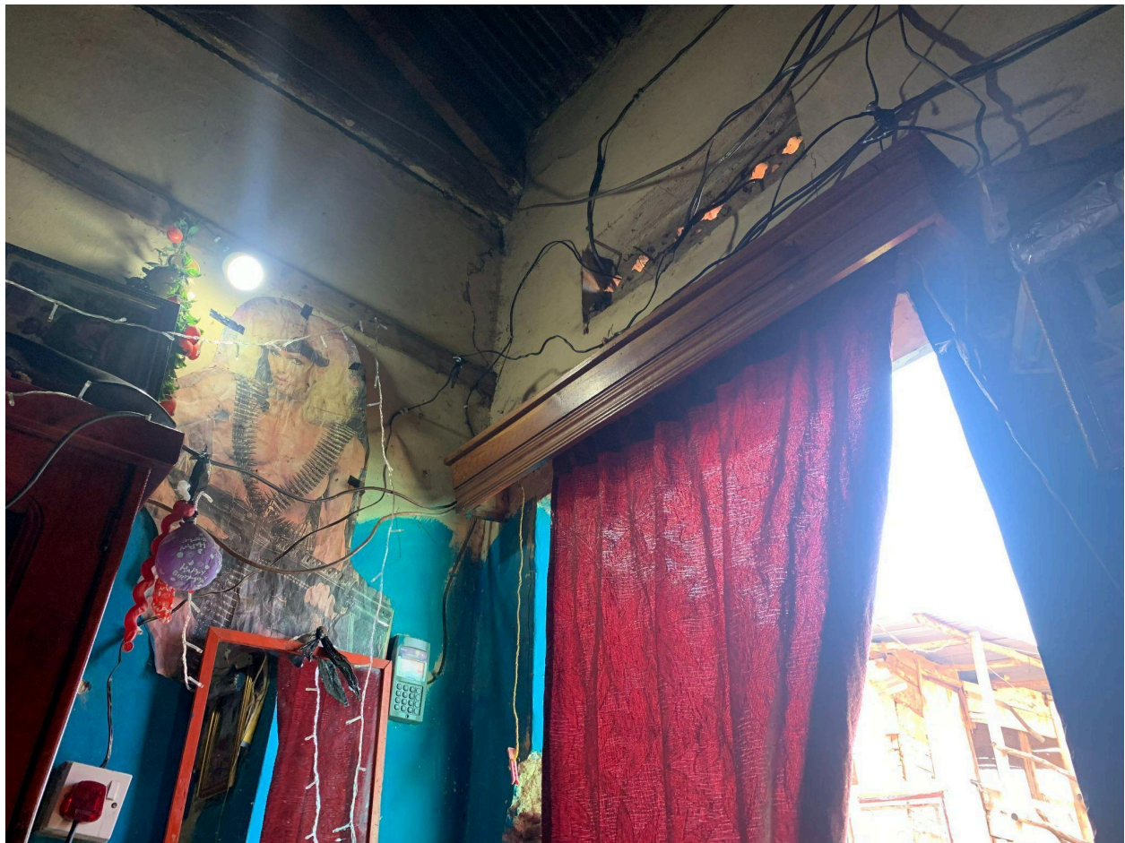
Photo 10. An example of improvised household wiring. This was the home of a family with two young children. The Yaka meter is visible to the left of the doorway but may be shared with nearby households. A family of this size uses electricity primarily for lighting, TV, phone charging, and other consumer electronics. Ironing and boiling water are other common household uses of electricity. The cables above the doorway show how wiring is extended ad hoc. Though the utility performs a wiring inspection as part of the registration process, internal wiring is usually added as money is available to purchase additional cables and outlets. Extension cables and power strips are often used as permanent wiring. The cost of internal wiring for a dwelling like this is around 30 USD. Because of this expense, it is common for renters to provide their own electrical wiring, which they usually remove and bring from their previous residence.
