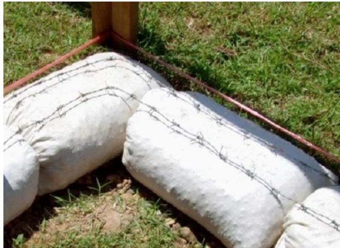
**Figure 5:** Barbed wire layout. Source: Geiger, O. (2015, September). *Earthbag Building Guide (Abridged and Adapted for Builders)*. Special Edition by Osho Tapoban Publications.
