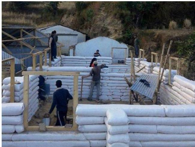
**Figure 3:** Earthbag Construction,
