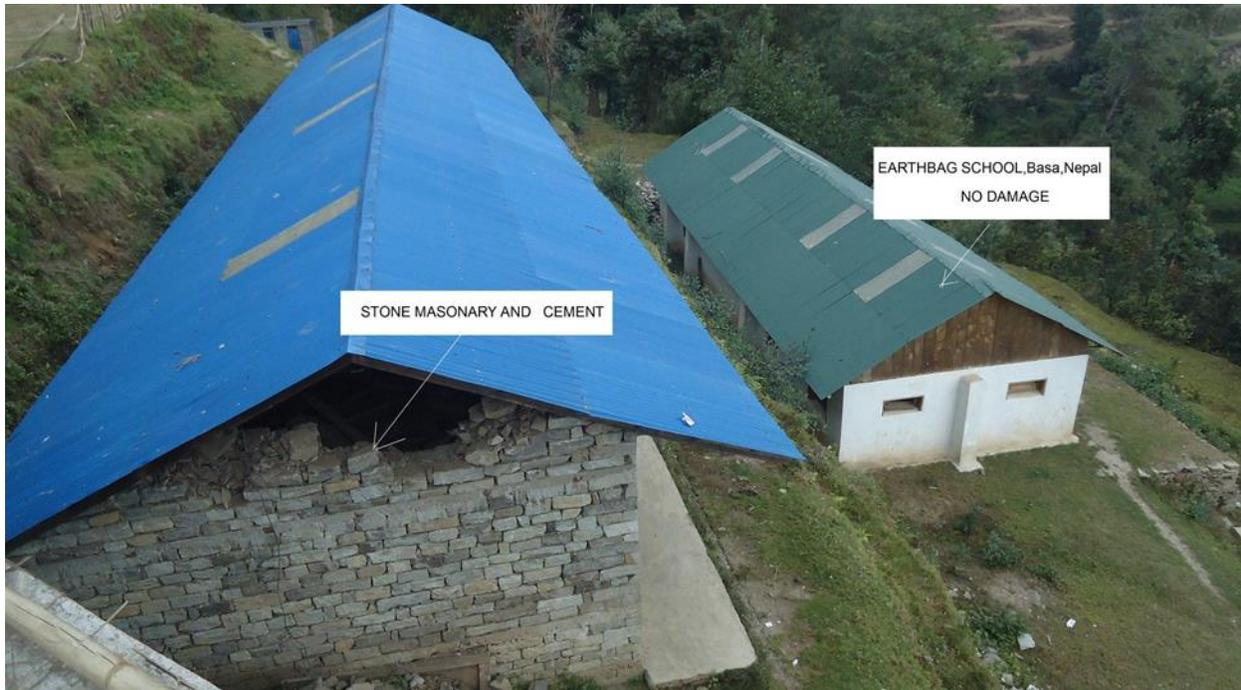
**Figure 8:** Earthbag School in Basa, Nepal (Edge of Seven, Small World) next to a damaged stone building
