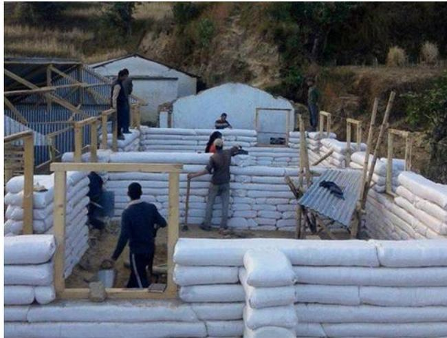
**Figure 3:** Earthbag Construction, Makwanpur, Nepal
