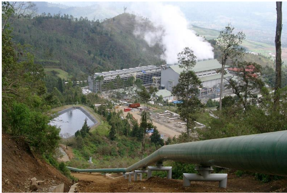
Figure 3: (Top) Schematic illustrating how a Flash Steam Geothermal Power Plant (the most common kind) works. Source: McDowell, R. (2006). "Indonesia sitting on geothermal power plant." NBCNEWS.com. (Bottom) Dajarat III Power Station, West Java, possessing 290 MW in capacity, rendering it the world's 10th largest geothermal plant as of 2013.
