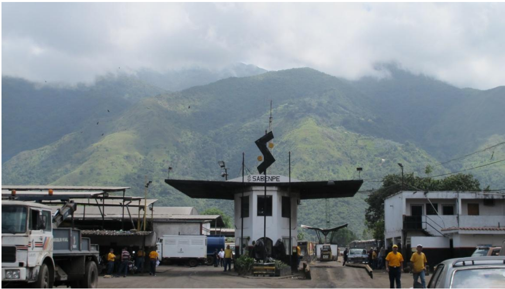
Figure 2: Entrance to Julian Blanco waste transference plant.
