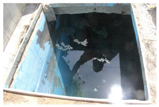
Photo 9: A reflection peering into a well during inspection; notice the peeling blue paint on the sides, another potentially contaminating factor.
