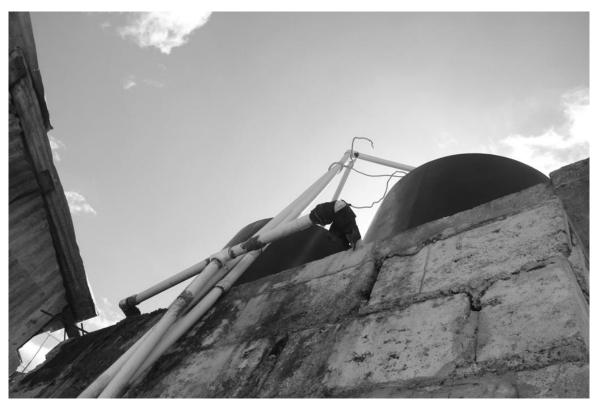
Photo 6: A typical "tinaco" water storage container sits atop a house; these devices often hold contaminated water.
