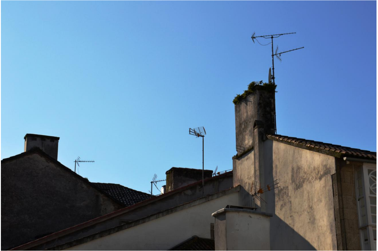
Figure 6: Roofs in Santiago.
