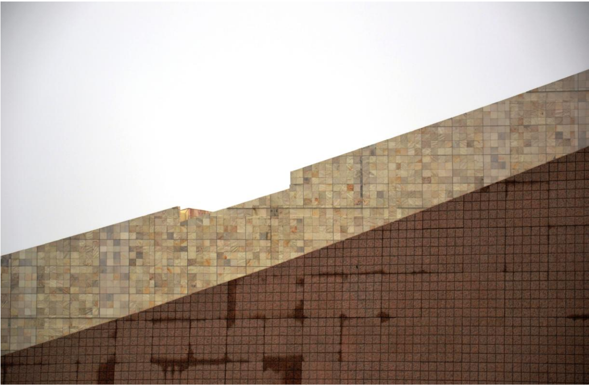
Figure 14: Roofs of the buildings that are, so far, the biggest built.
