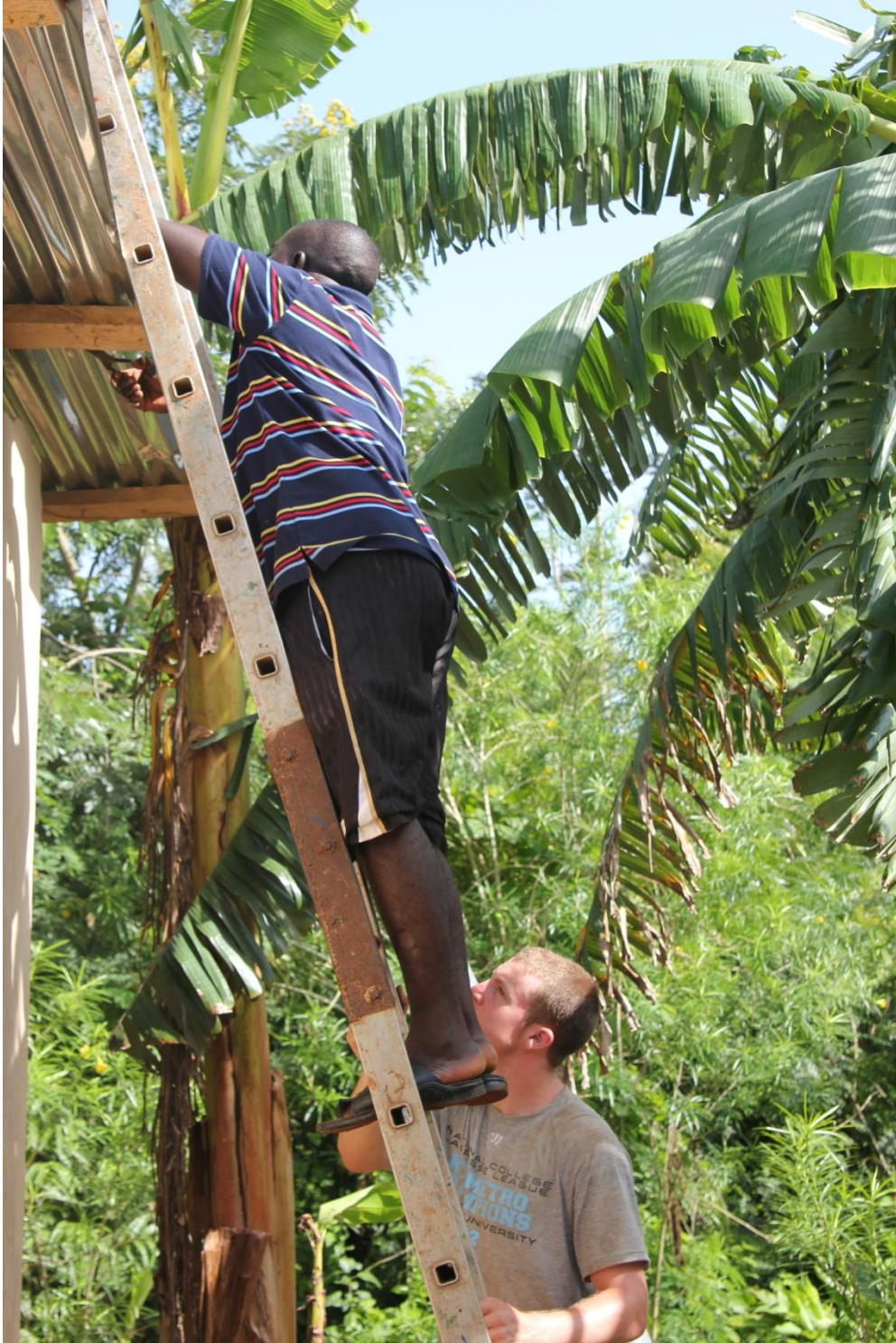
Figure 3: A Columbia student stabilizes a ladder while an Obodan man prepares the latrine roof for ventilation installation.
