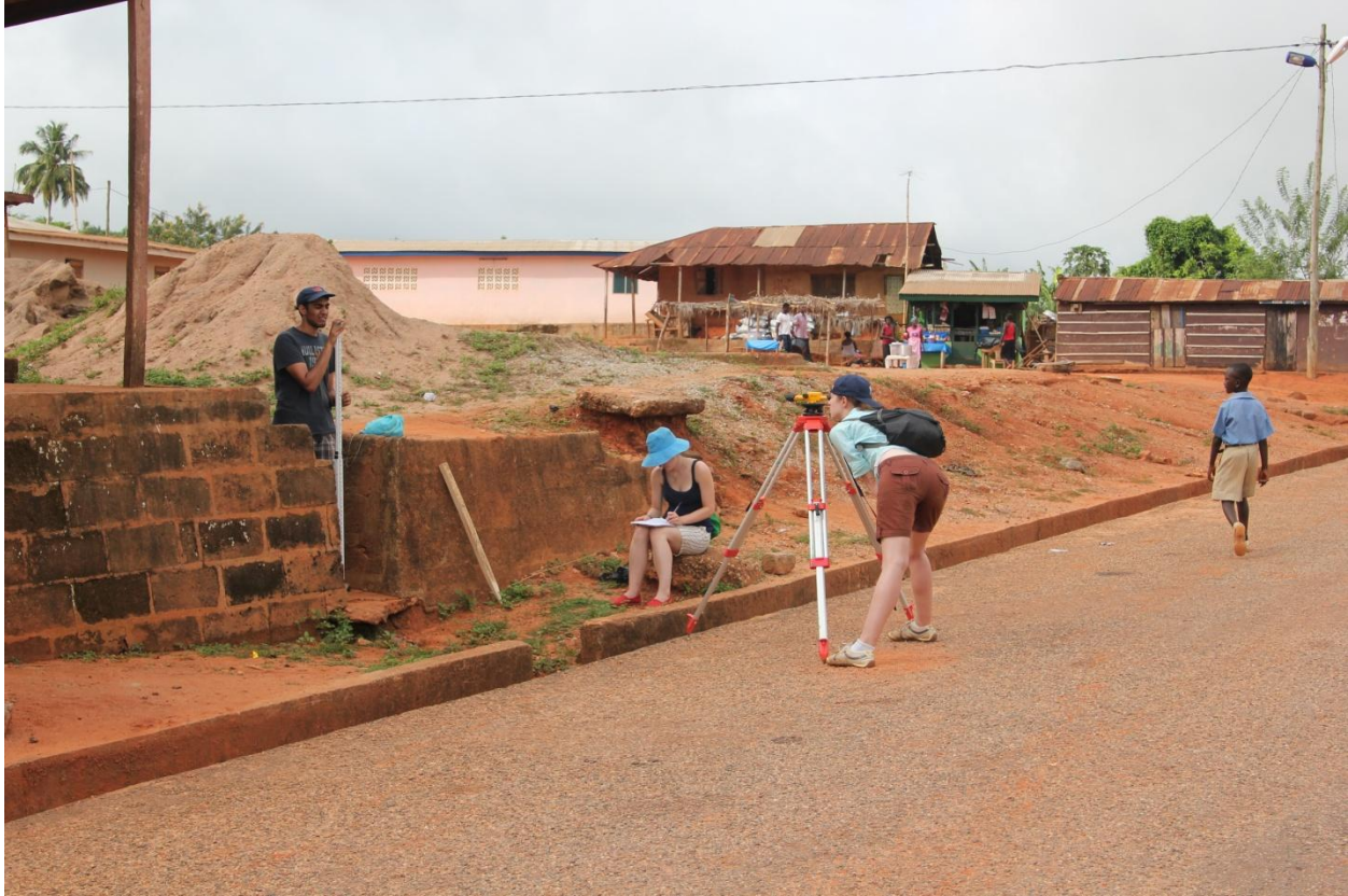
Figure 4: Columbia students take surveying data along a proposed pipeline for the water distribution system.
